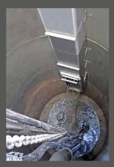
The Bar Screen is installed into the station, facing the water inlet, against the station's wall.
