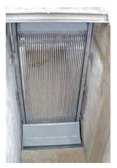
The Bar Screen is installed into the channel, across the flow, discharging the waste either upstream or downstream depending on the technical requirements.
